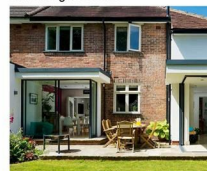
Full height window to rear bedroom
