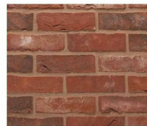
Red facing brickwork
